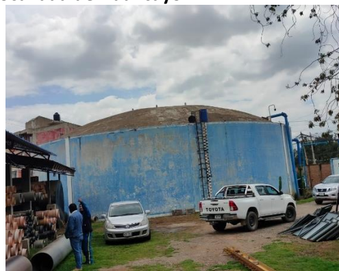
Reservorios San Antonio 3,000 m 3
